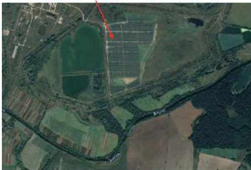
Fig. 7. Solar power plant on the hydro dump No. 1
